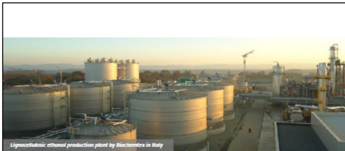
Lignocellulosic ethanol production plant by Biochemtex in Italy
